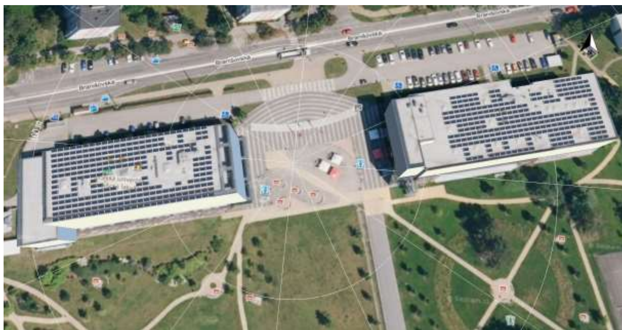
Image overview, 3D design, Rectorate building and FAR USB and USB Academic Library. Photo: Project study of the technological solution
